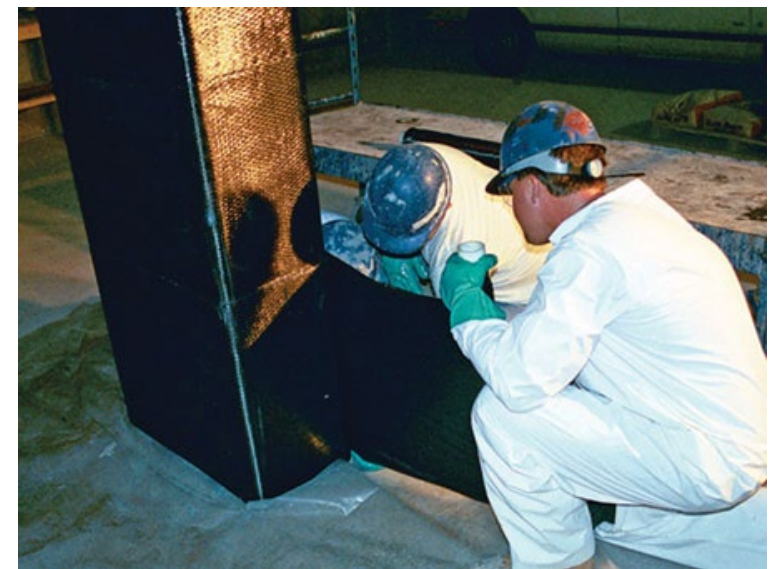
Concrete column reinforcement wrap
