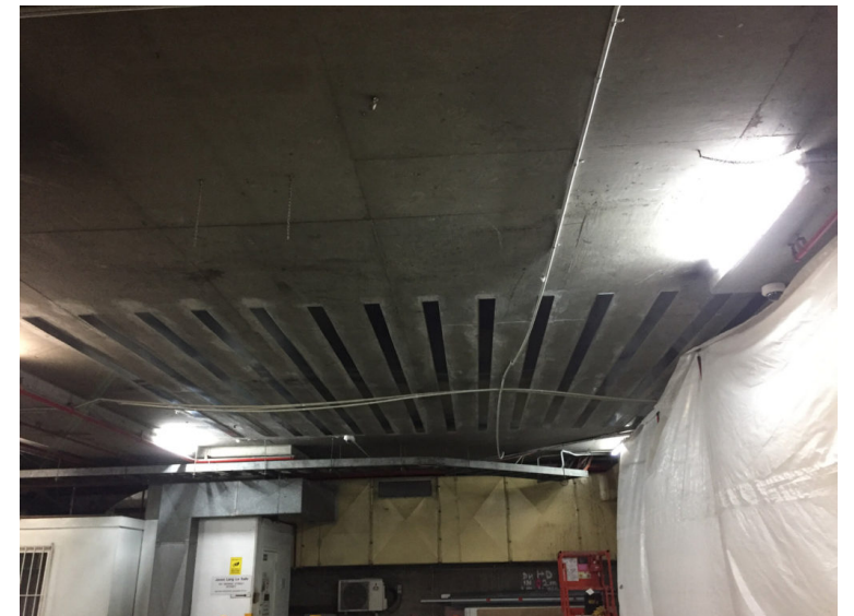
Slab reinforcement strips
