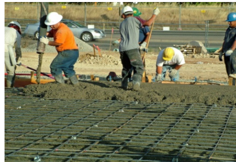
Modern highways are composites of concrete and steel re-bar
