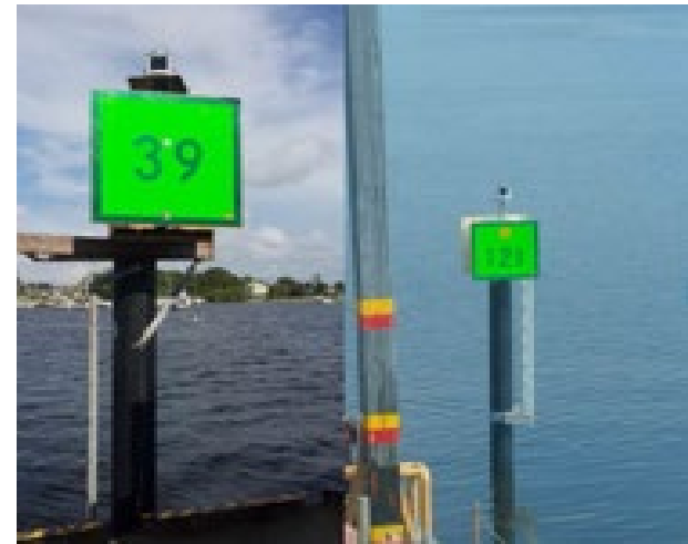
Navigation Aids with FRP Piles
