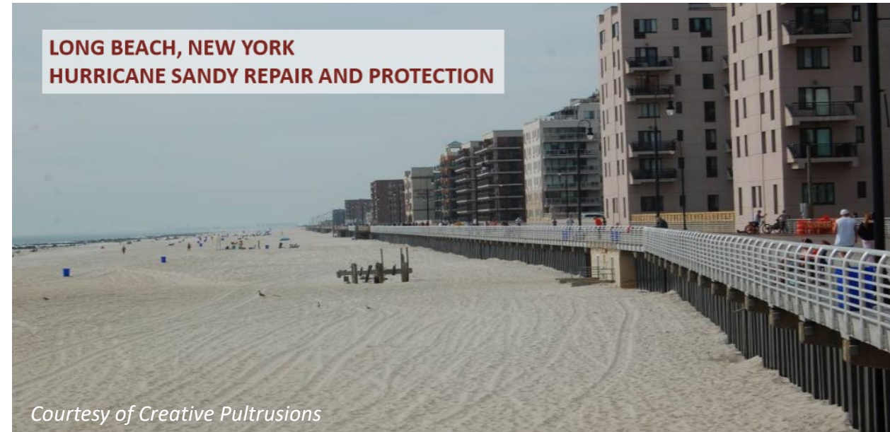
Seawall in New York built after Hurricane Sandy
