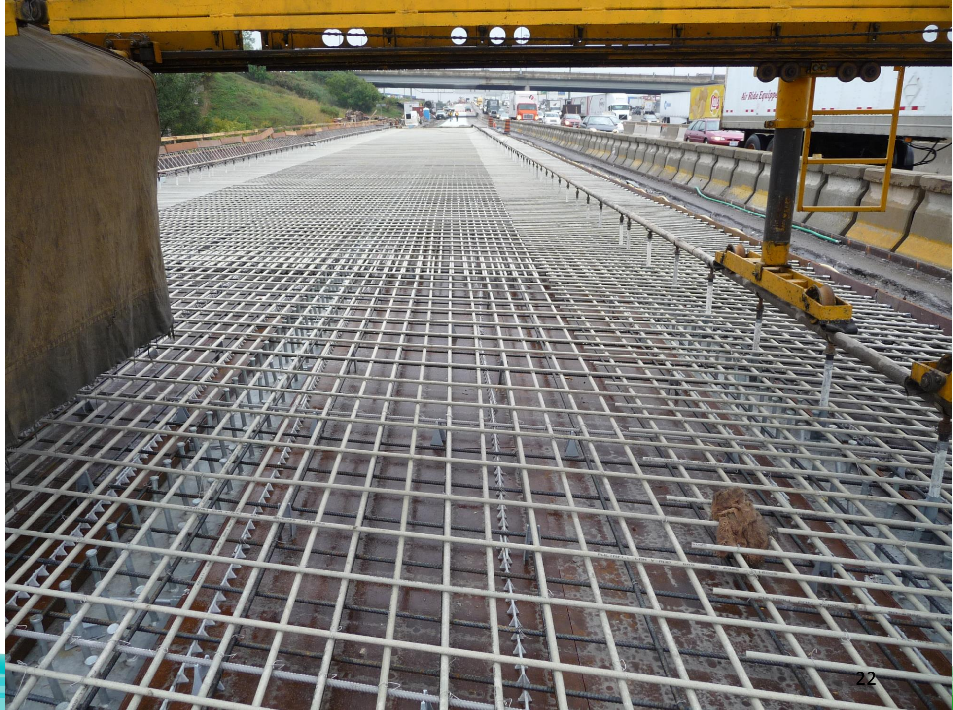
MTO 2009-2020 (Hwy 401 in Toronto) multiple cast in place deck structures
