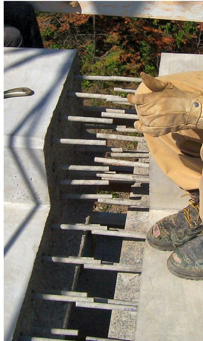
Rainy Lake - 2006, MTO NW Region Pre-cast panels decks
