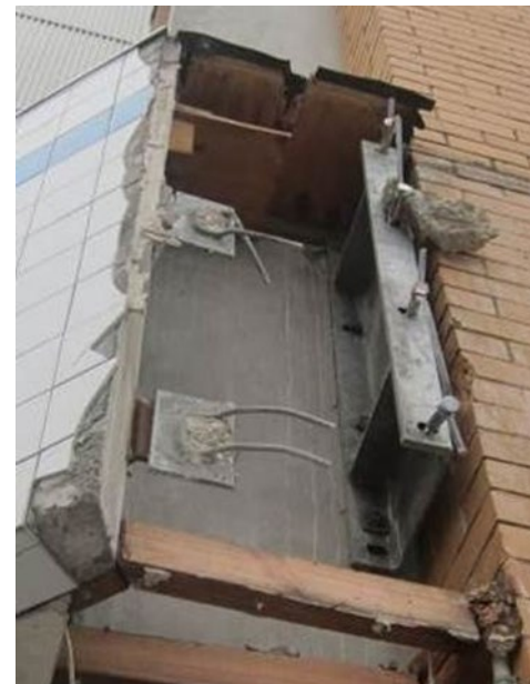
Pre-cast panel failure following seismic activity
