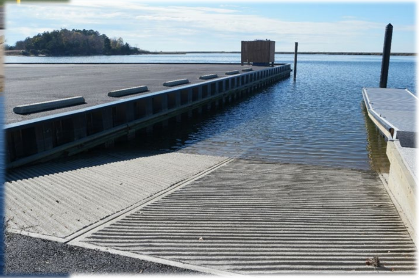
COLBOURNE CREEK BOAT RAMP - MD DNR - MARION STATION, MD
