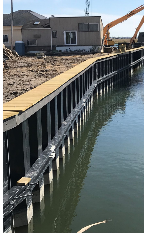
Tie Rods with Anchors
