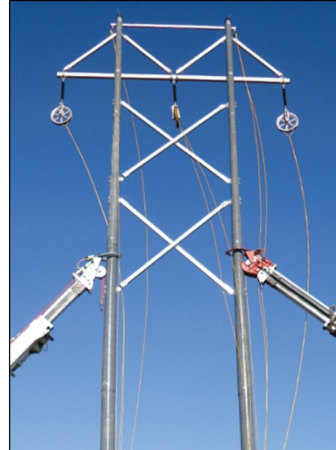
2003 – FRP Transmission H-Frames up to 345kV Introduced
