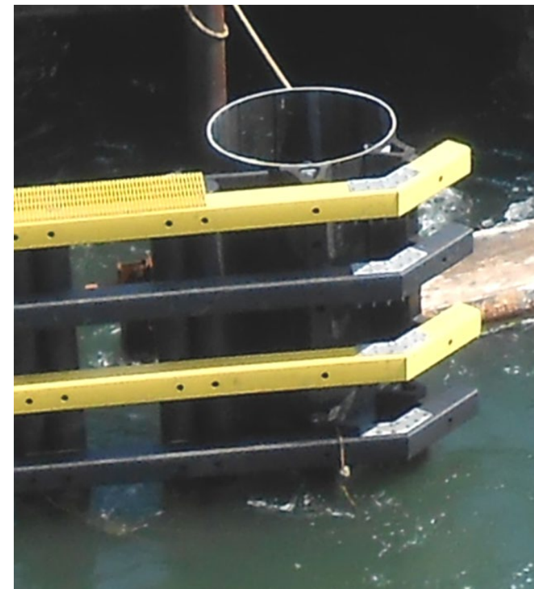
AMTRAK BRIDGE FENDER NIAN TIC RIVER
