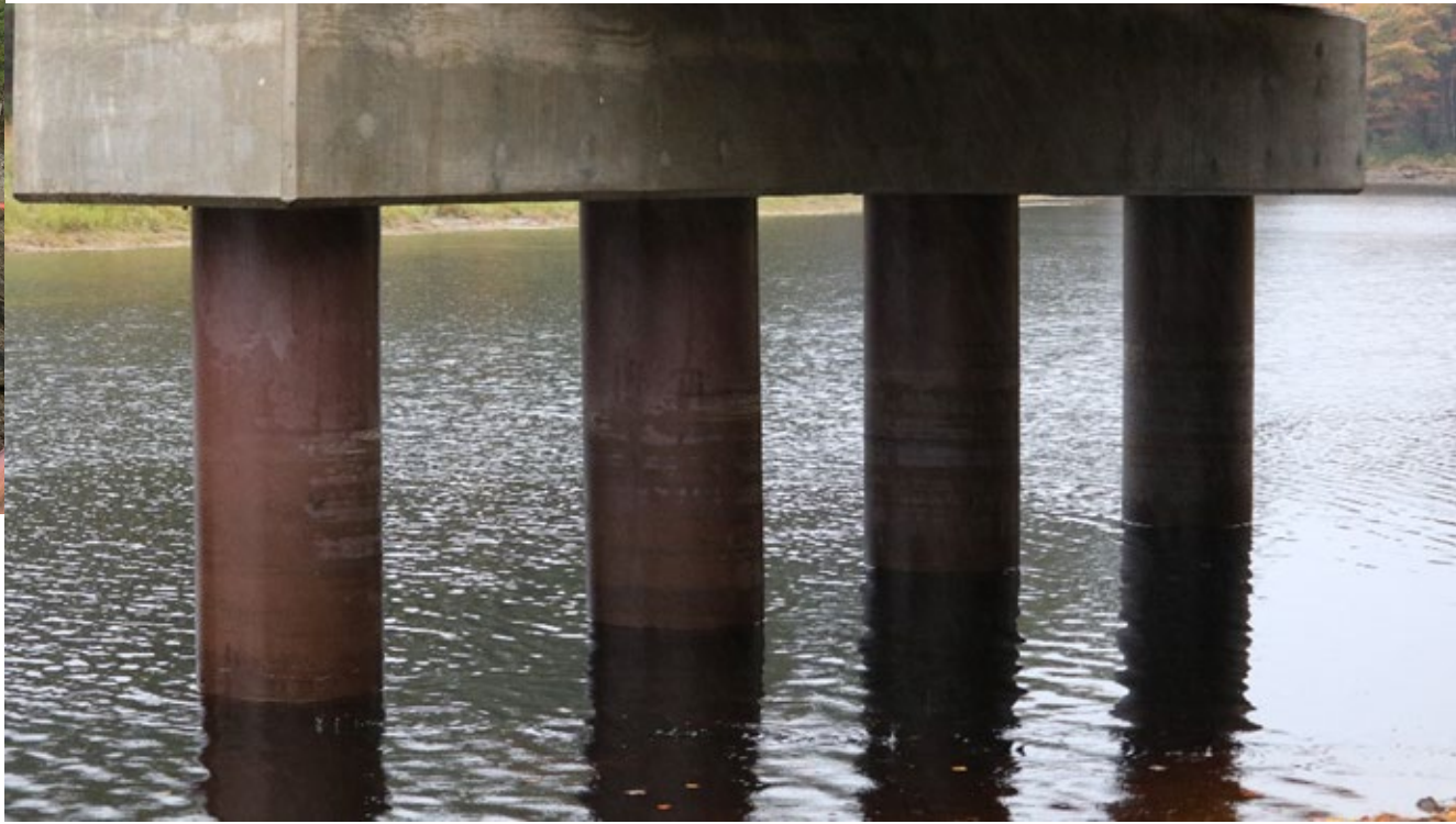
MAINE DOT ~ GOODWIN BRIDGE
