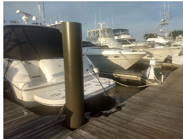
Floating Dock Piles
