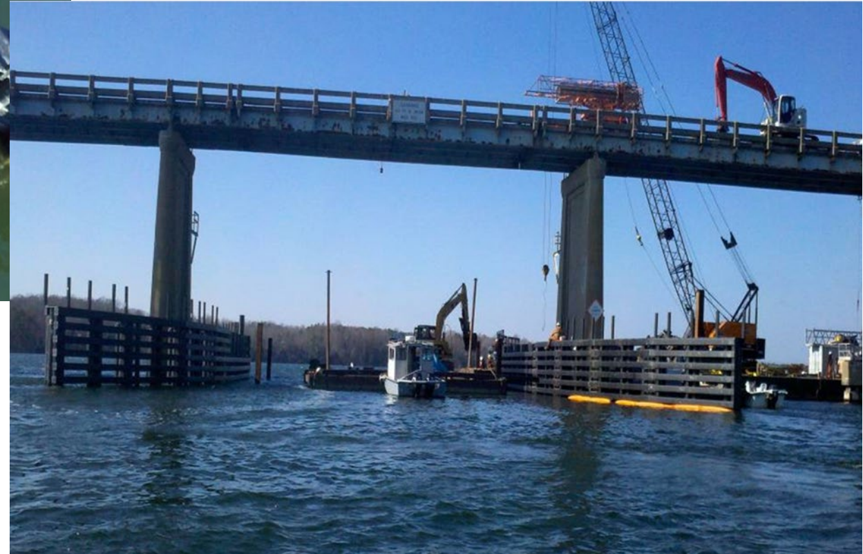
TWIGG BRIDGE ~ VIRGINIA DOT
