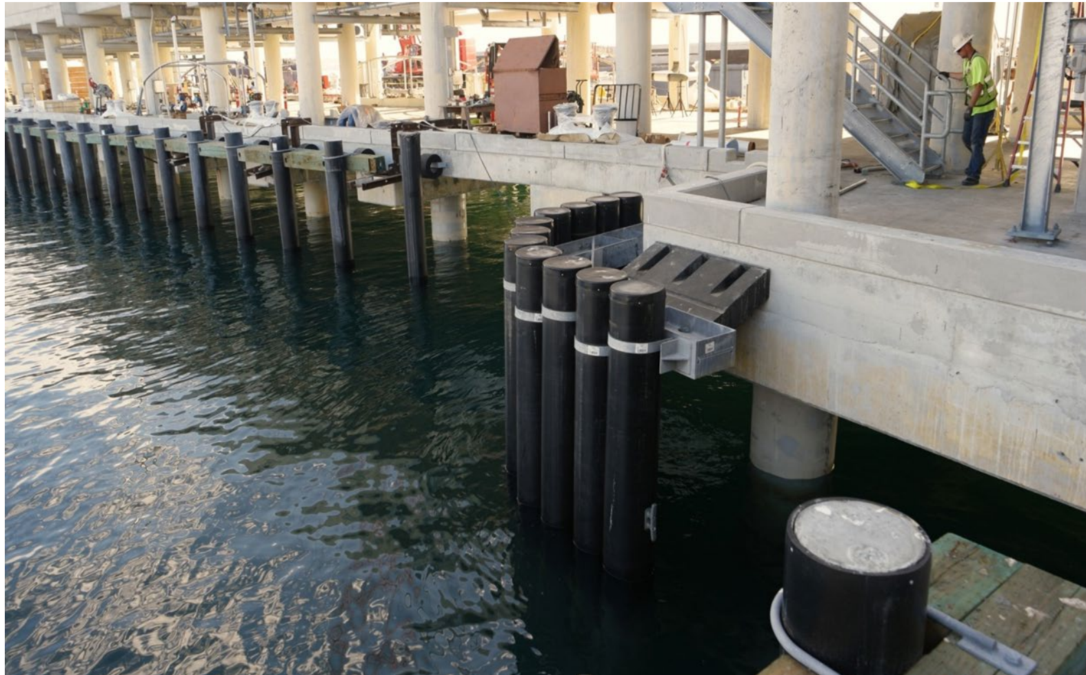
FUEL PIER - USN POINT LOMA
