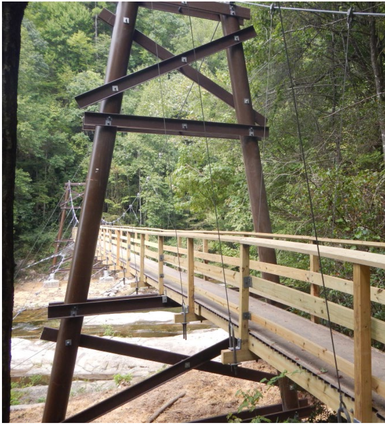
Duke Energy Toxaway Bridge ~ Gorges State Park, Sapphire, NC
