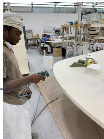
Finisher spraying a patch
