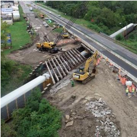
Anthony Wayne Trail Bridge
