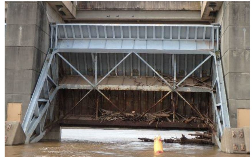
Downstream View of Tainter Gate
