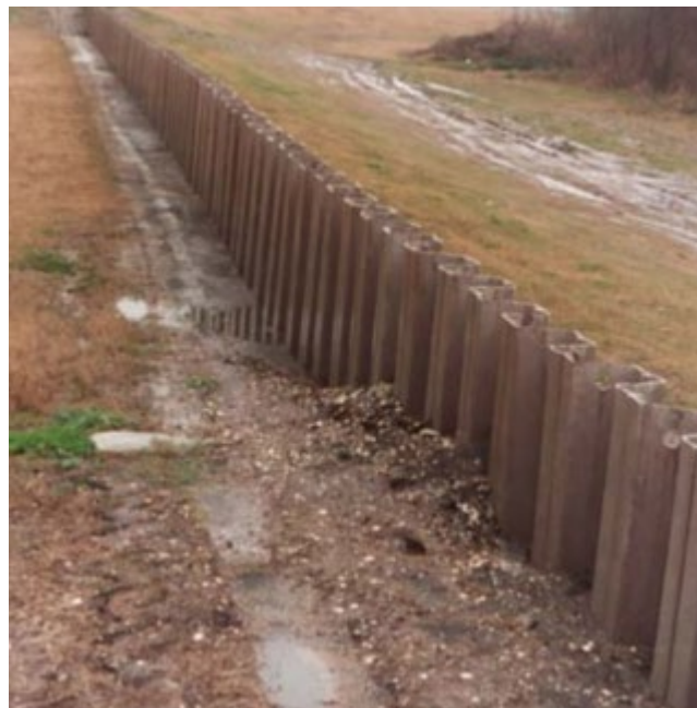
PVC sheet pile floodwall installed 1998 in Jefferson Parish, Louisiana
