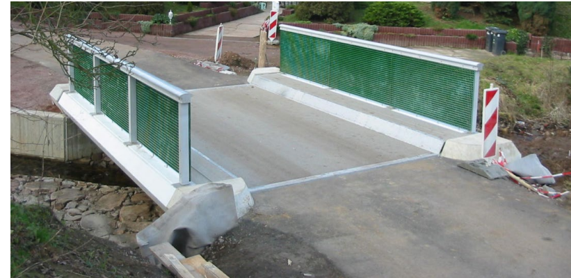
GFRP-bridge after installation; Source: Fiberline A/S
