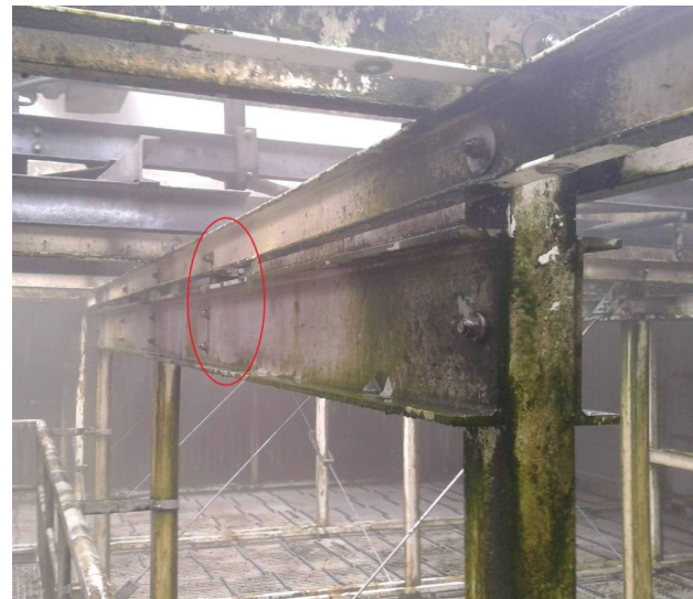
Structure of cooler tower with GFRP-profiles; Source: Fiberline A/S
