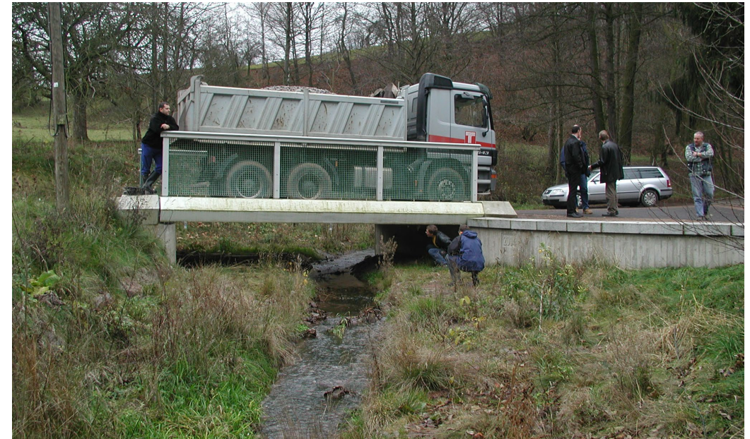
GFRP-bridge: After installation with Truck (weight approx. 20 t); Source: IMA
