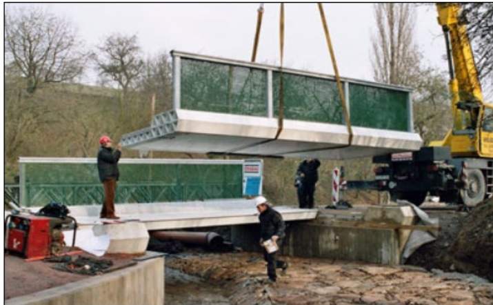
GFRP-bridge: During installation; Source: Fiberline A/S
