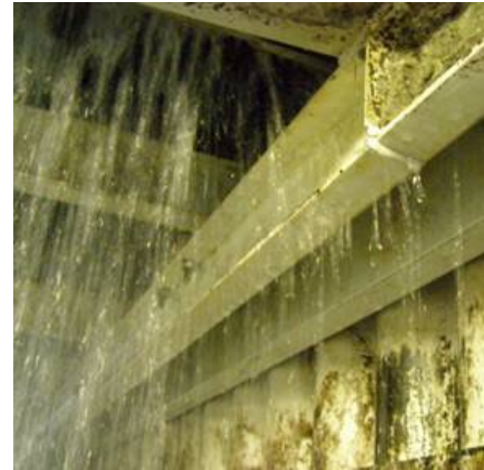
GFRP profiles in cooling tower
