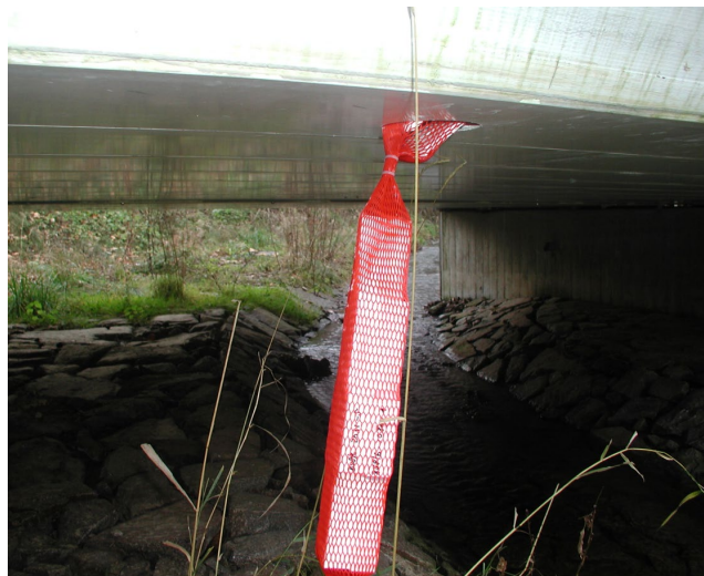
Witness samples inside the bridge; Source: IMA
