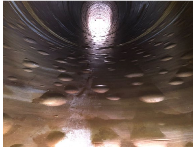
Bubbles inside clean gas channel (CGC)
