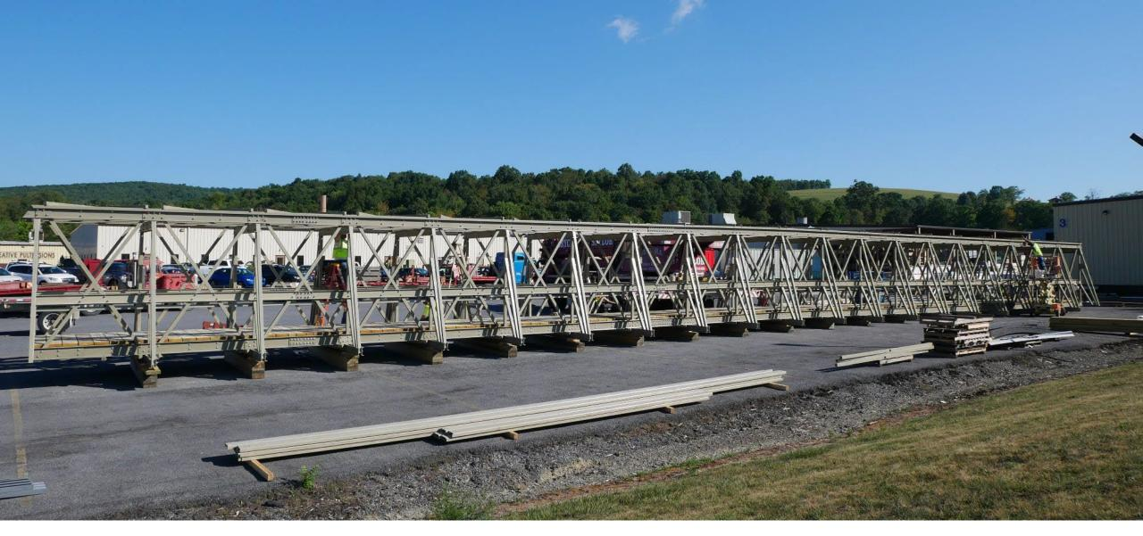
Bottom chord length of bridge is 152'-2"; 148'-8" c/c bearings bridge length
