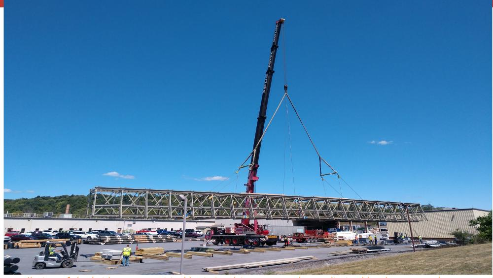
Crane Lift for Installation of the bridge was a critical logistics driver. Bermuda was limited by the cranes that are available on the island. As part of test program, the lift was simulated the Bermuda pick in the CCG yard. Each lift utilized eight pick points. Equipment here shown was sent to Bermuda, except the crane. The lift required was 20ft in the air.
