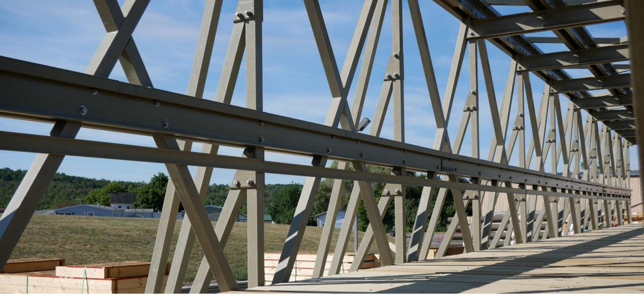
8'-3" wide (c/c truss) box structure cross section – 20 bays @ 7'-7 3/4" ± spacing
