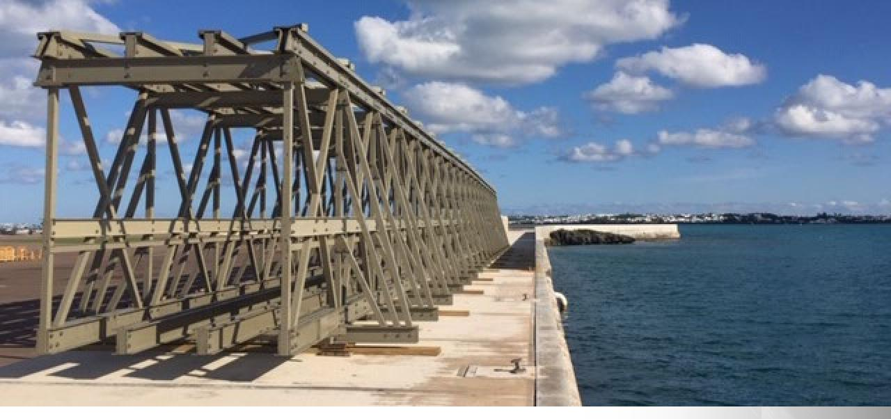
Bridge assembled on pier in Bermuda, ready to be ferried to site.
