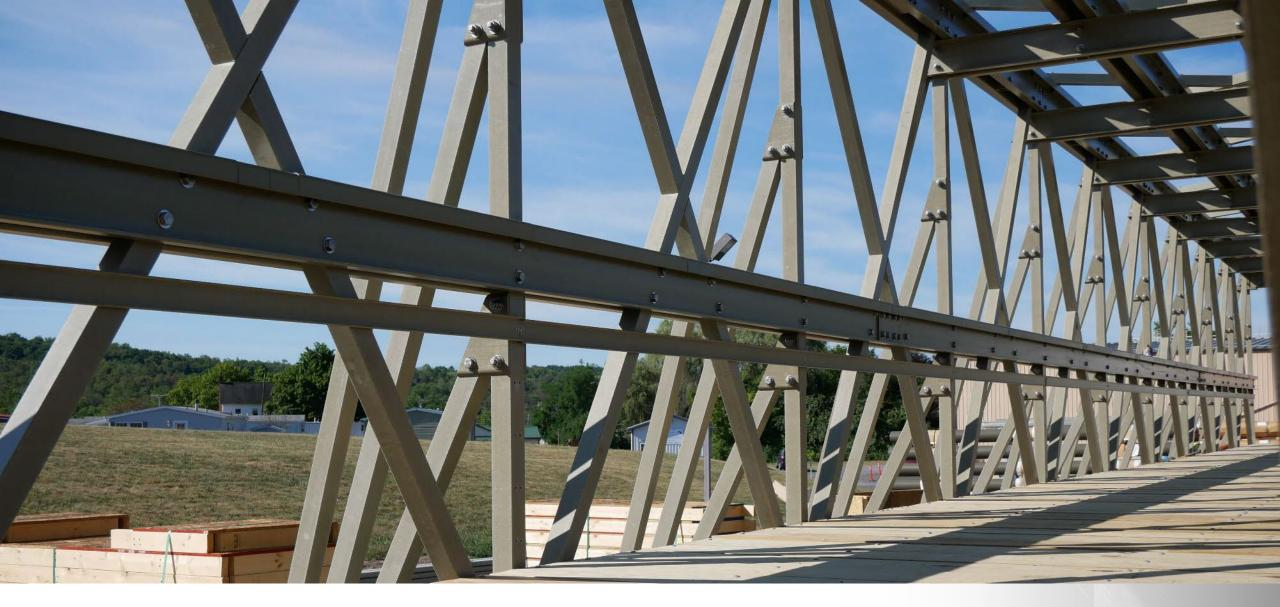
8'-3" wide (c/c truss) box structure cross section – 20 bays @ 7'-7 <sup>3</sup>/<sub>4</sub>" ± spacing
