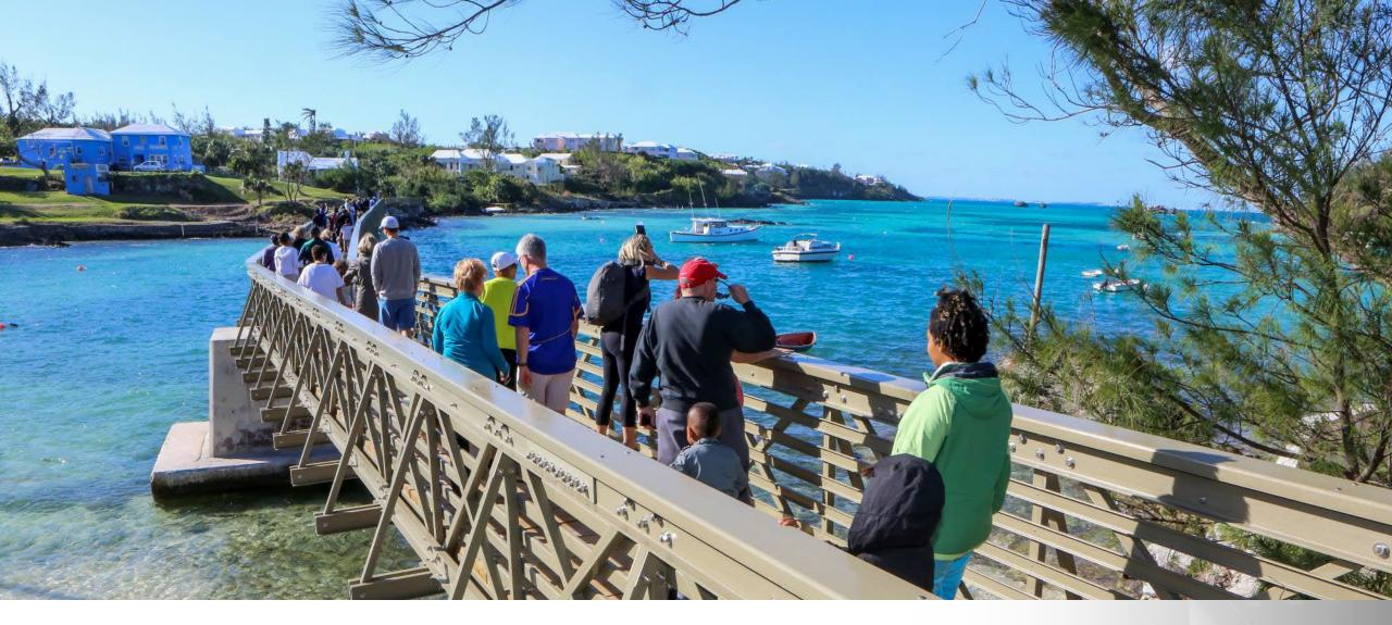
In 2017, Friends of Bermuda Railway Trail tapped Creative Composites Group to provide a fiber reinforced polymer (FRP) pedestrian bridge from its E.T. Techtonics line. We've previously installed six bridges. There was one major hurdle.
