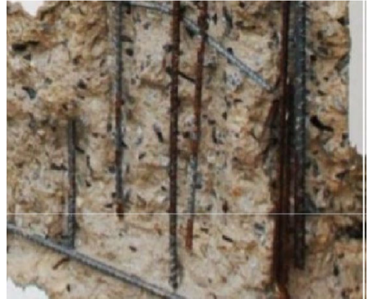
Chloride induced corrosion
