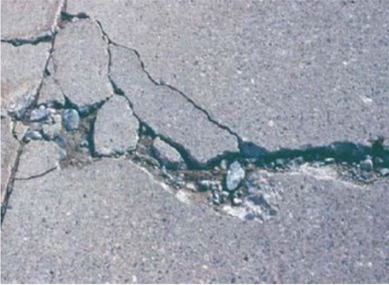
Freeze/thaw due to water ingress
