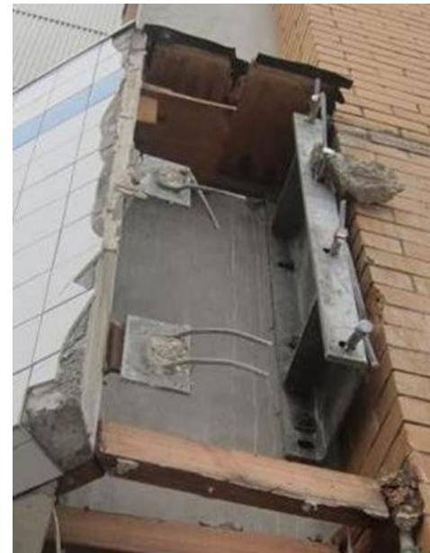
Pre-cast panel failure following seismic activity
